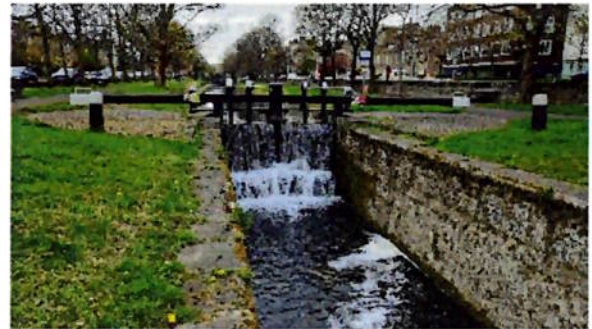
Plate 8.2 Lock C2 (Mount Street Bridge) – another barrier to linear otter passage along the Grand Canal
