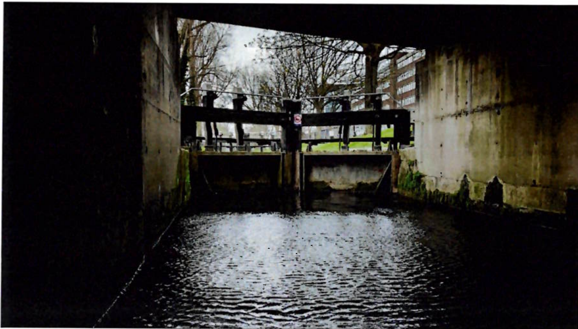
Plate 4.1 The Grand Canal at lock C1 (Macquay's Bridge) presents a significant barrier to otter movement given an absence of steps or ledges and a fall of approx. 1.8m
