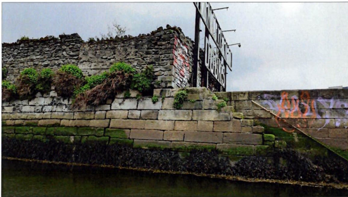
Plate 4.4 The quay steps on the River Dodder estuary which appear to be the main commuting/access route for otters moving between estuarine habitat and the Grand Canal Basin
