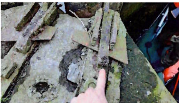
Plate 8.3 Otter spraint site recorded on the C1 lock structure (Macquay's Bridge)
