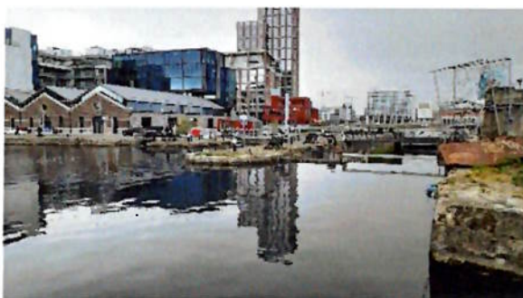
Plate 8.15 View of Camden Lock (right), Buckingham Lock (centre) and Westmoreland Lock (left) from the graving docks
