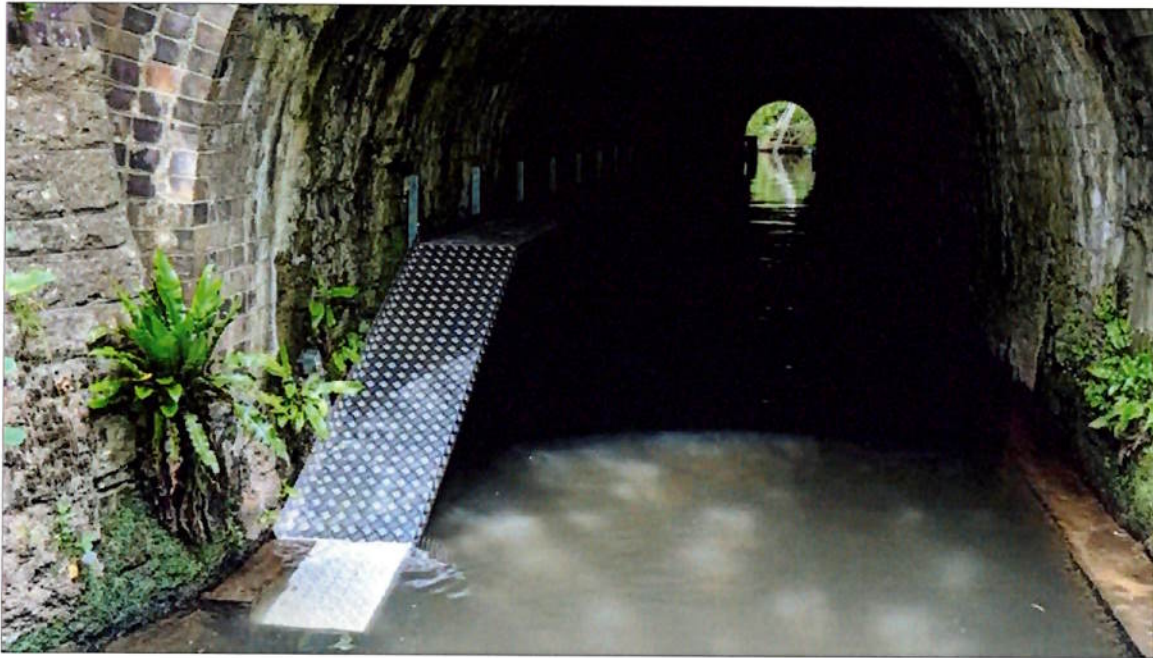
Plate 5.4 Example of best practice bolt-on steel mammal shelf/ledge for otter passage under culverts (source: Landmarc Environmental Engineering, UK)
