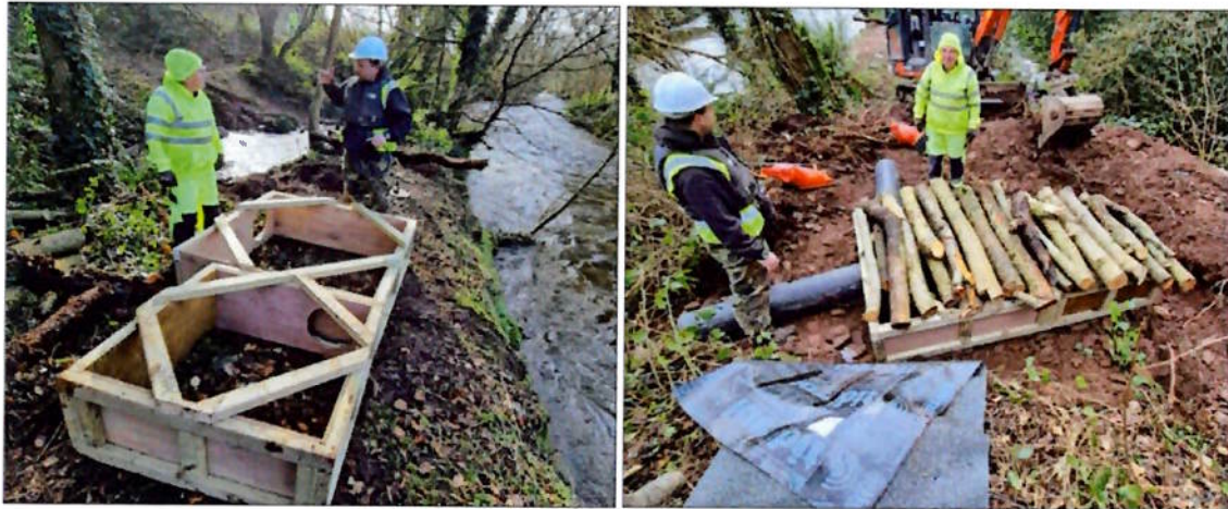
Plate 5.1 Example of a double-chambered artificial otter holt designed and installed by Triturus Environmental Ltd. on the Glashaboy River, Co. Cork in 2021 (left: box structure, right: natural log roof) Macklin, R. (2022)
